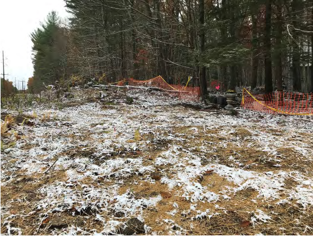
Fig 7: Restored and straw mulched access route southwest of Str. 89. Viewing south. (10-30-20)
