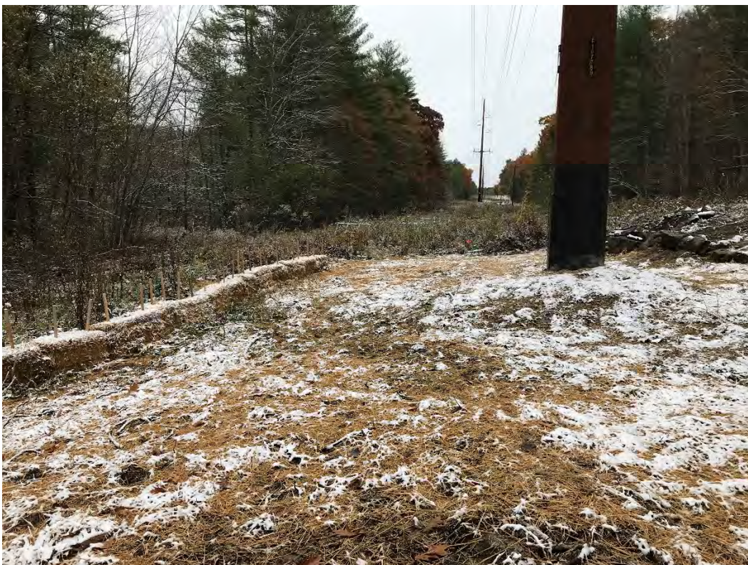
Fig 6: Restored and straw mulched Str. 89 work area. (10-30-20)
