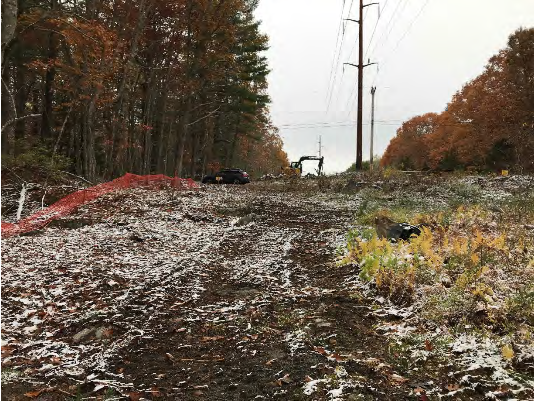
Fig 9: Access leading from wetland DW22 to Longmarsh Rd. Viewing northwest. (10-30-20)
