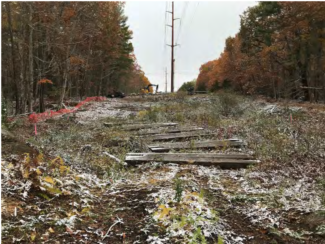
Fig 8: Matted access route across wetland DW22. Viewing southeast. (10-30-20)
